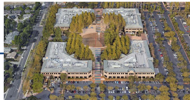
Google Quad on Whisman Road. Source: Google Earth 2016
