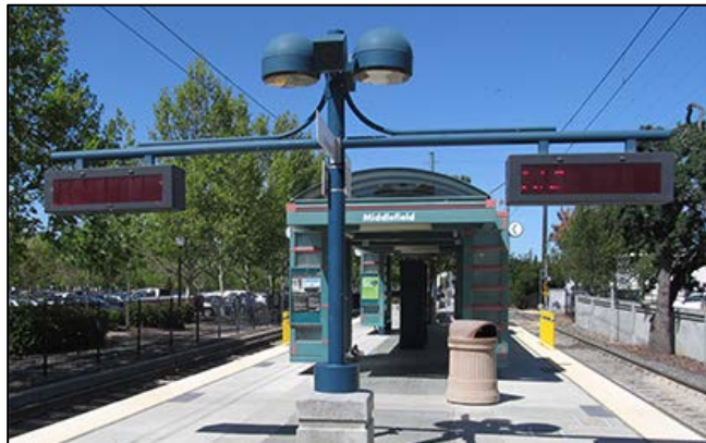
Middlefield Light Rail Station.
