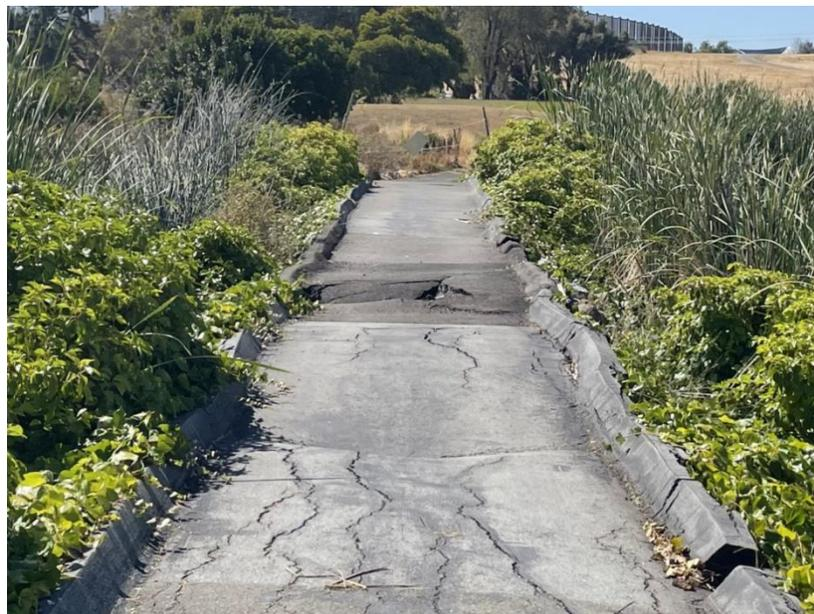
Photo 2. Closeup of existing deterioration Bridge #25.
