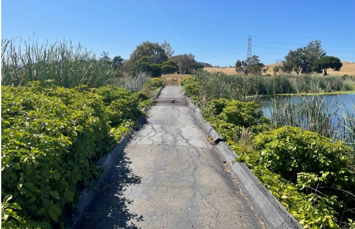
Photo 1. View of Existing City Bridge #25 looking southeast across the top of the existing deteriorated causeway.<sup>1</sup>
