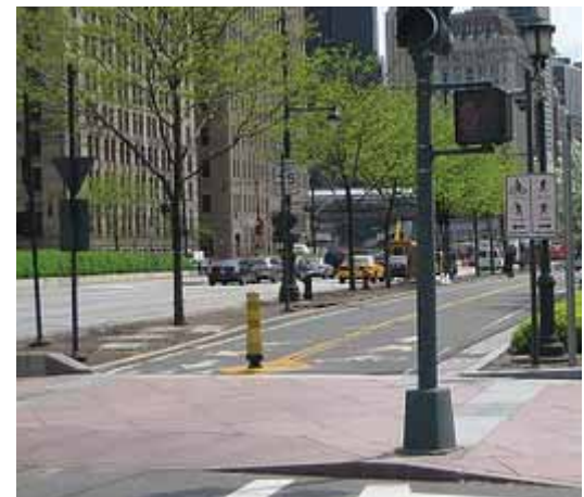
Separated lanes could be located adjacent to the roadway, rather than inside the parkway given the existing width of the Hetch Hetchy right-of-way.
