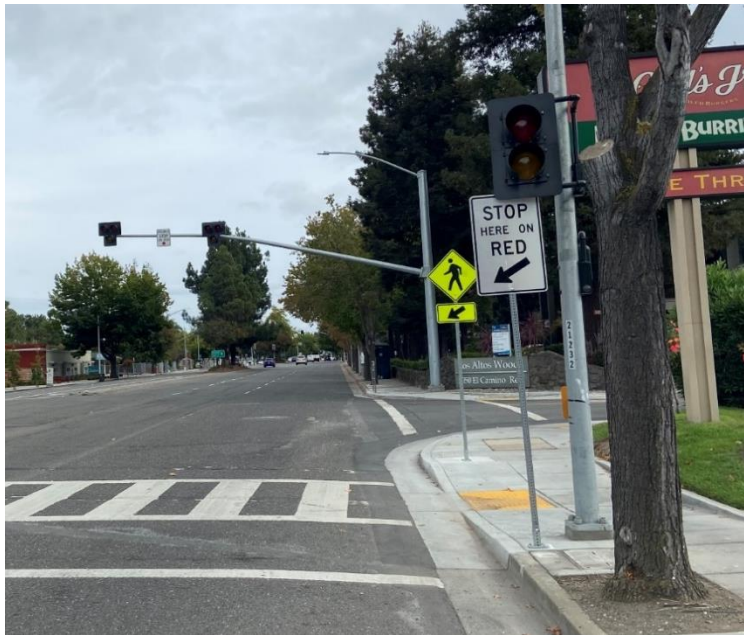
Figure 3—PHB at Distel Circle and El Camino Real, Mountain View/Los Altos Border
