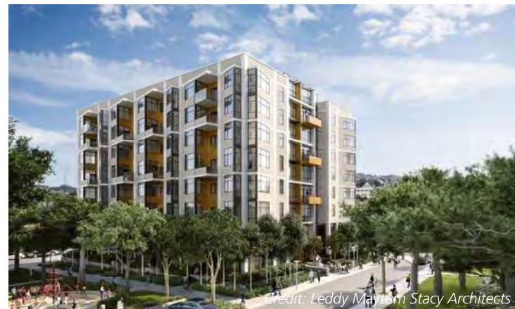
7m. Articulate residential building façades with smaller-scale increments than office building façades. Use windows, balconies, and bays for residential buildings to reflect the scale of residential rooms rather than open office floors. Taller residential buildings should have fewer building façade increments than mid-rise residential buildings.
