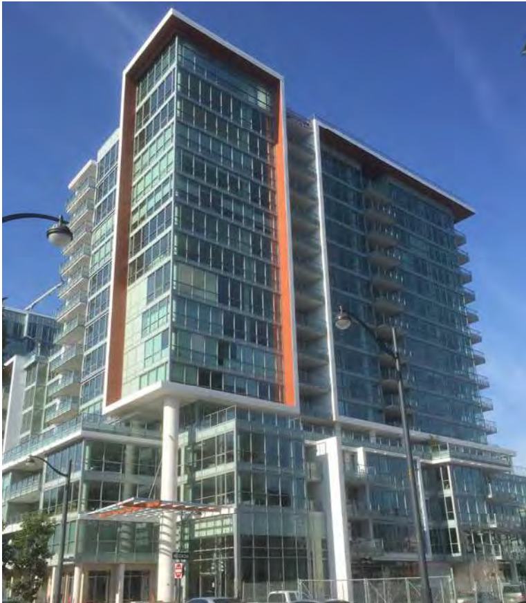
7k. Use building organization and construction to derive their scale and articulation rather than surface ornamentation.
