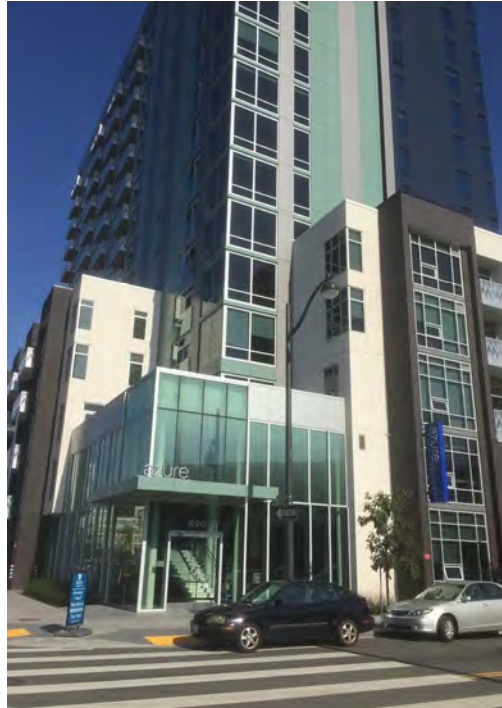
4h. Integrate high-rise (above 95 feet) residential building forms, into the design of the structure through massing, materials, and detailing to ensure the high-rise form is connected to the building base or podium.
