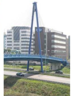
Rivium GRT Guideway, Netherlands
