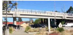
VTA Hamilton Station Viaduct Guideway
