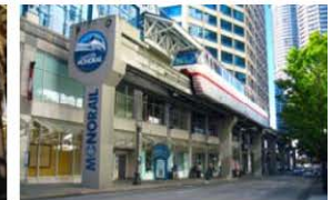
Seattle Monorail Guideway
