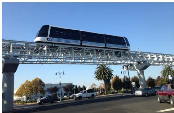
Doppelmayr Cable Car: Cable Liner (Oakland, CA)
