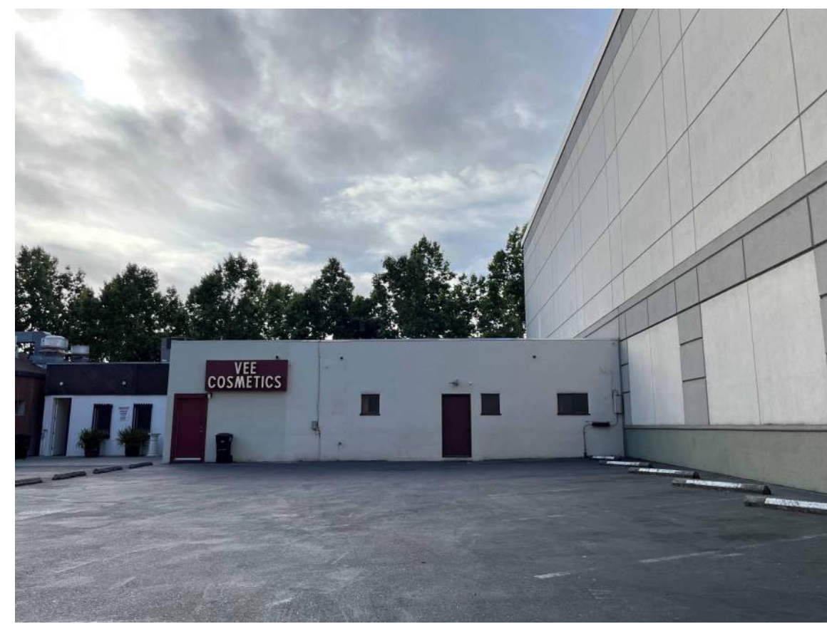
(E) REAR BUILDING VIEW SHOWING ADJACENT BUILDINGS
