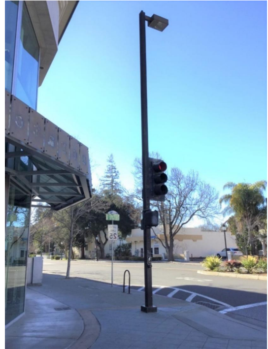
Figure 11 - Existing Shoebox Style Flood Light
