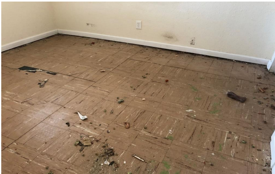
Figure 6: Floorboard of Rear Structure
