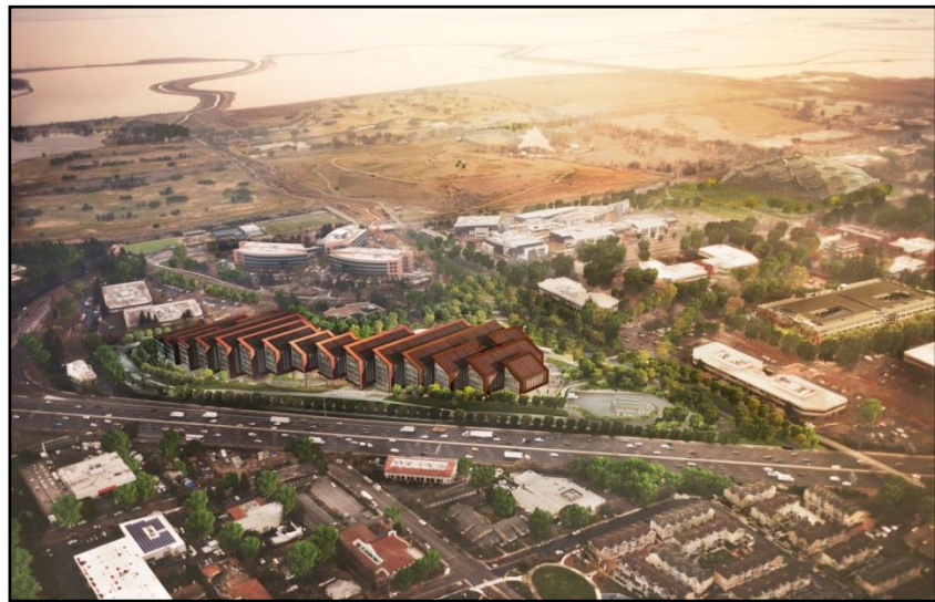
Aerial View of Project
