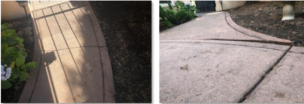
Figure 2: Sidewalk Cracks
