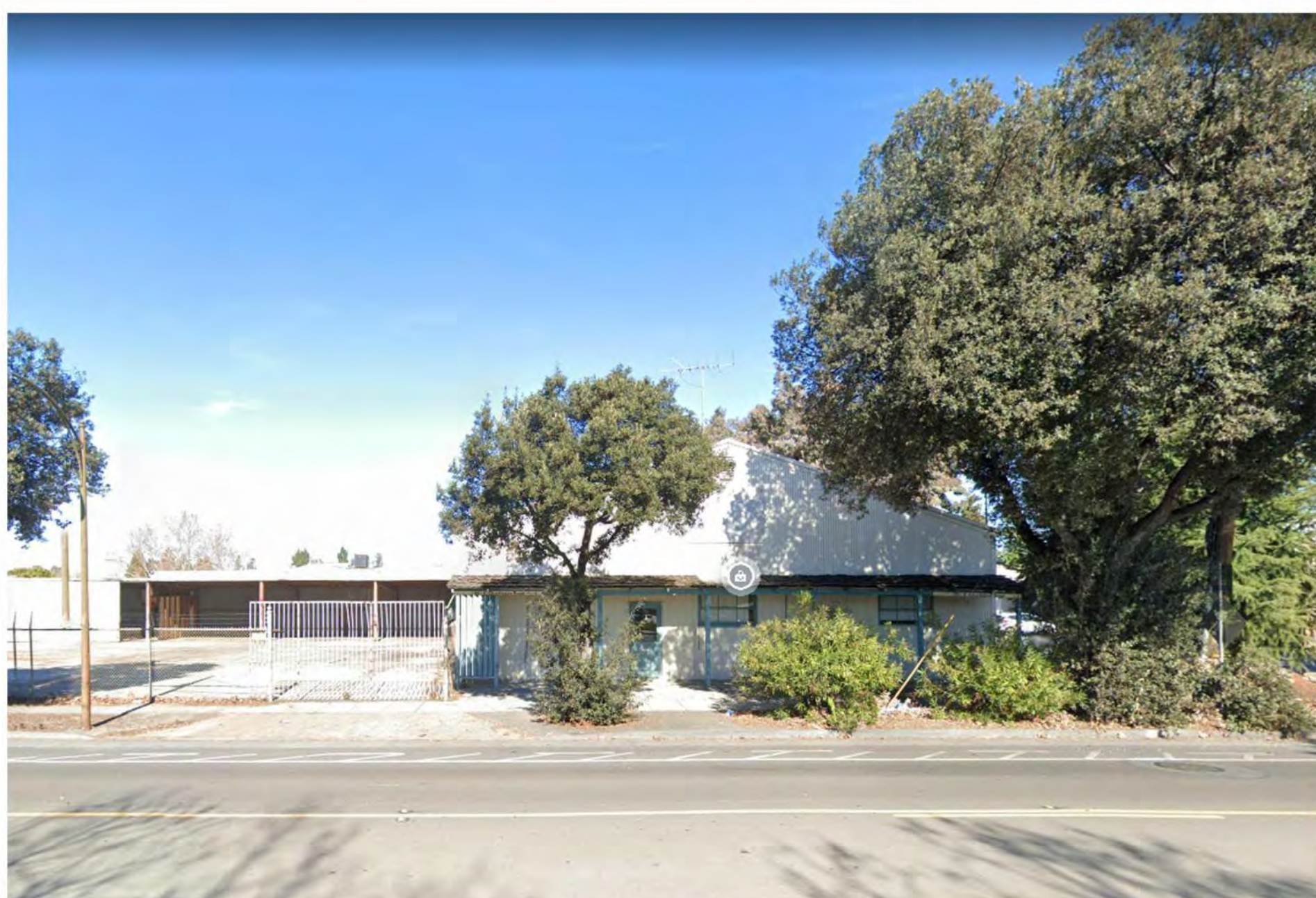
6. VIEW NORTH ON CHARLESTON, NEIGHBORING INDUSTRIAL BUILDING
