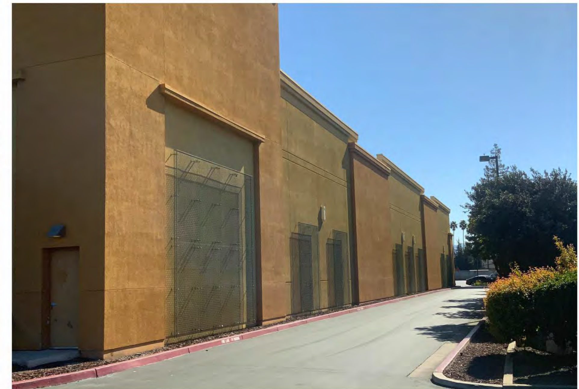
8. BUILDING M1 FIRE ACCESS/LOADING ACCESS ROAD
