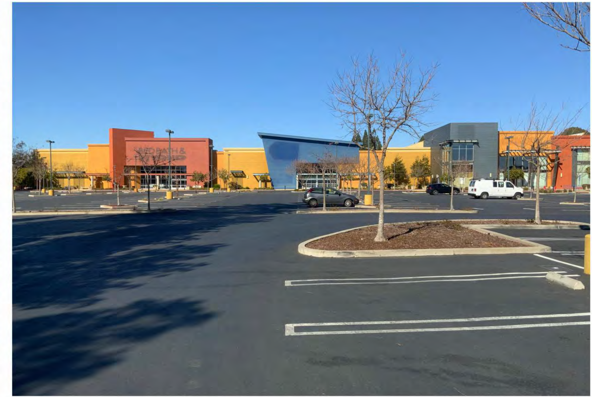
5. VIEW OF BUILDING SOUTH ELEVATION FROM CHARLESTON
