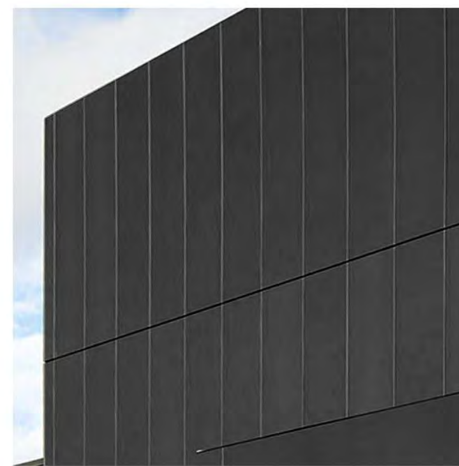
B1-4 ALUMINUM PANEL RAINSCREEN NORTHCLAD OR EQ. ACM RAINSCREEN PANEL, CONCEALED FASTENERS, LEXUS BRONZE
