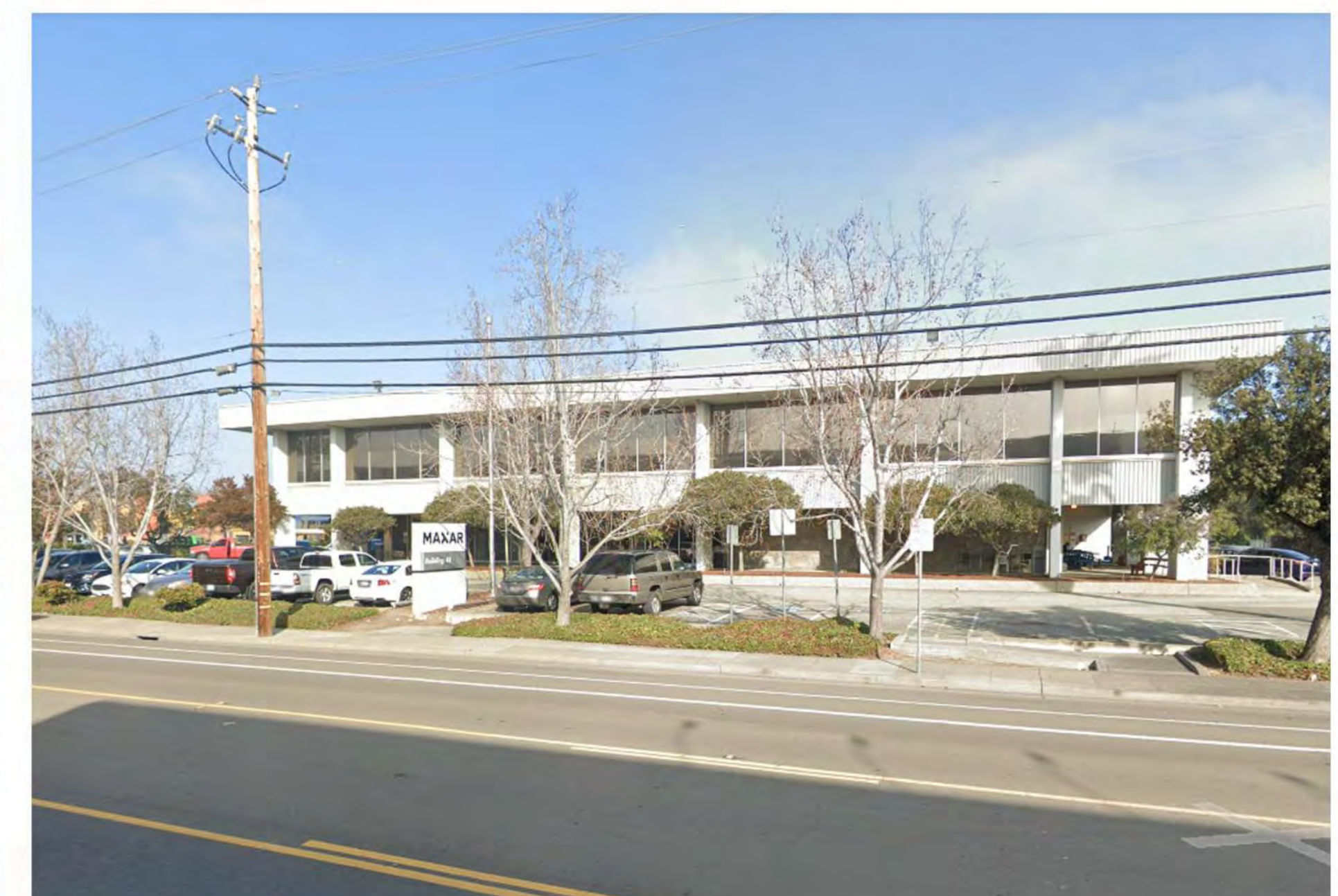
8. VIEW NORTH ON CHARLESTON, NEIGHBORING INDUSTRIAL BUILDING
