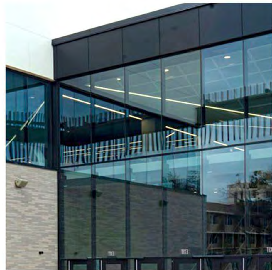
C1-2 BUTT JOINT GLASS SYSTEM MULLIONS SIT BEHIND GLAZING WITH TINE, WALTERS & WOLF OR EQ., PAINTED DARK GREY
