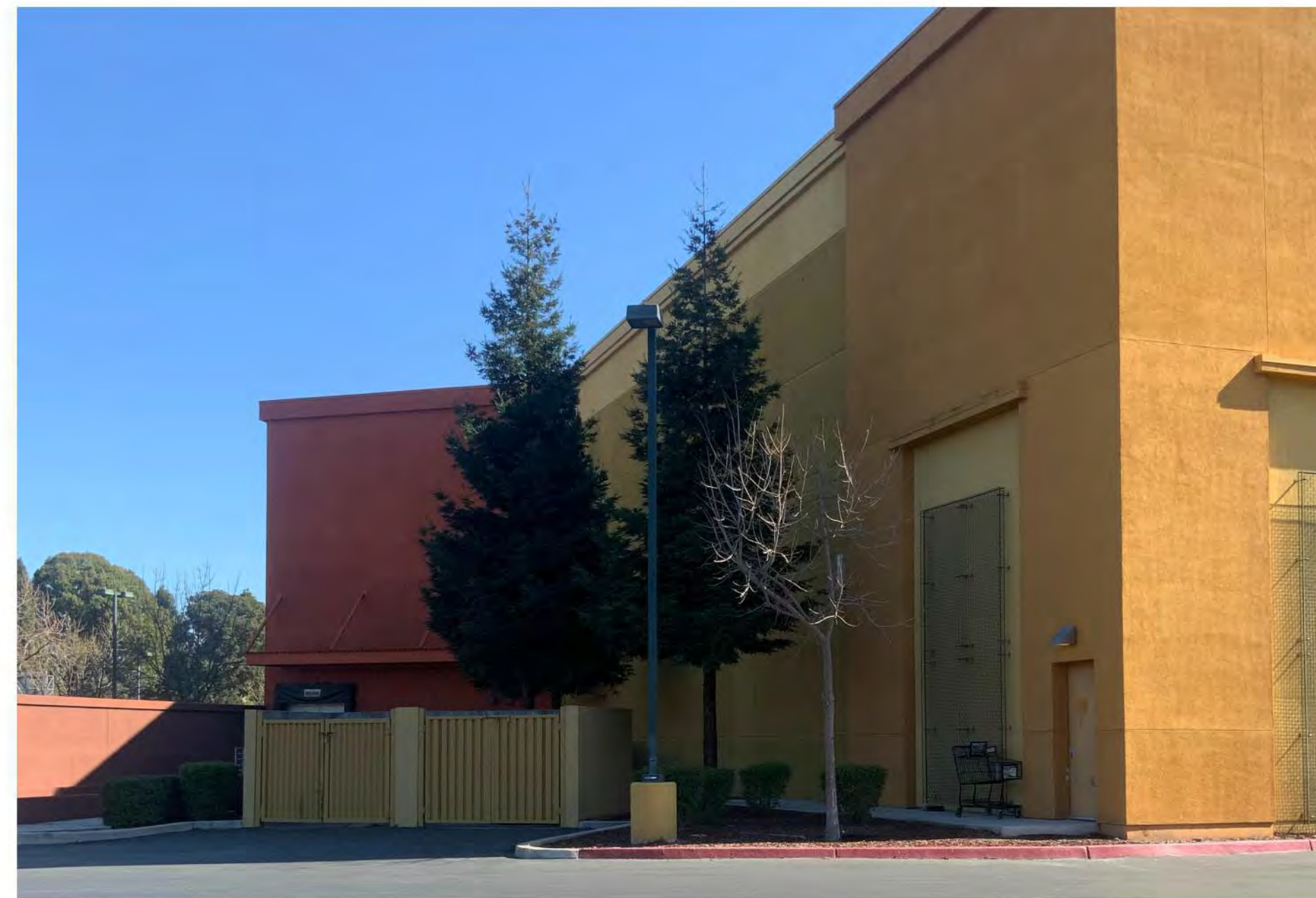
7. M1 LOADING FROM REAR ACCESS ROAD
