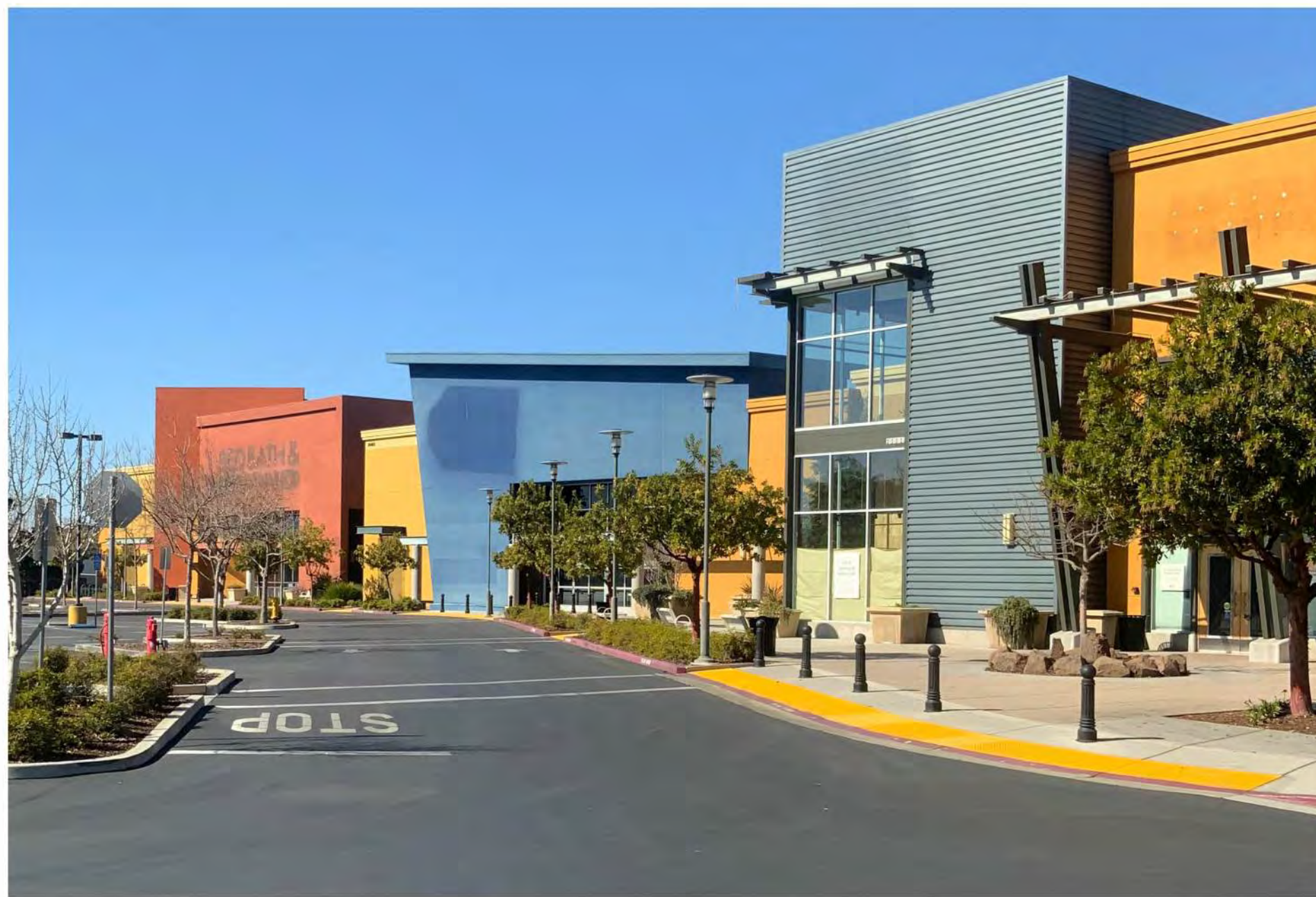
4. VIEW OF BUILDING SOUTH ELEVATION, M1 - M3
