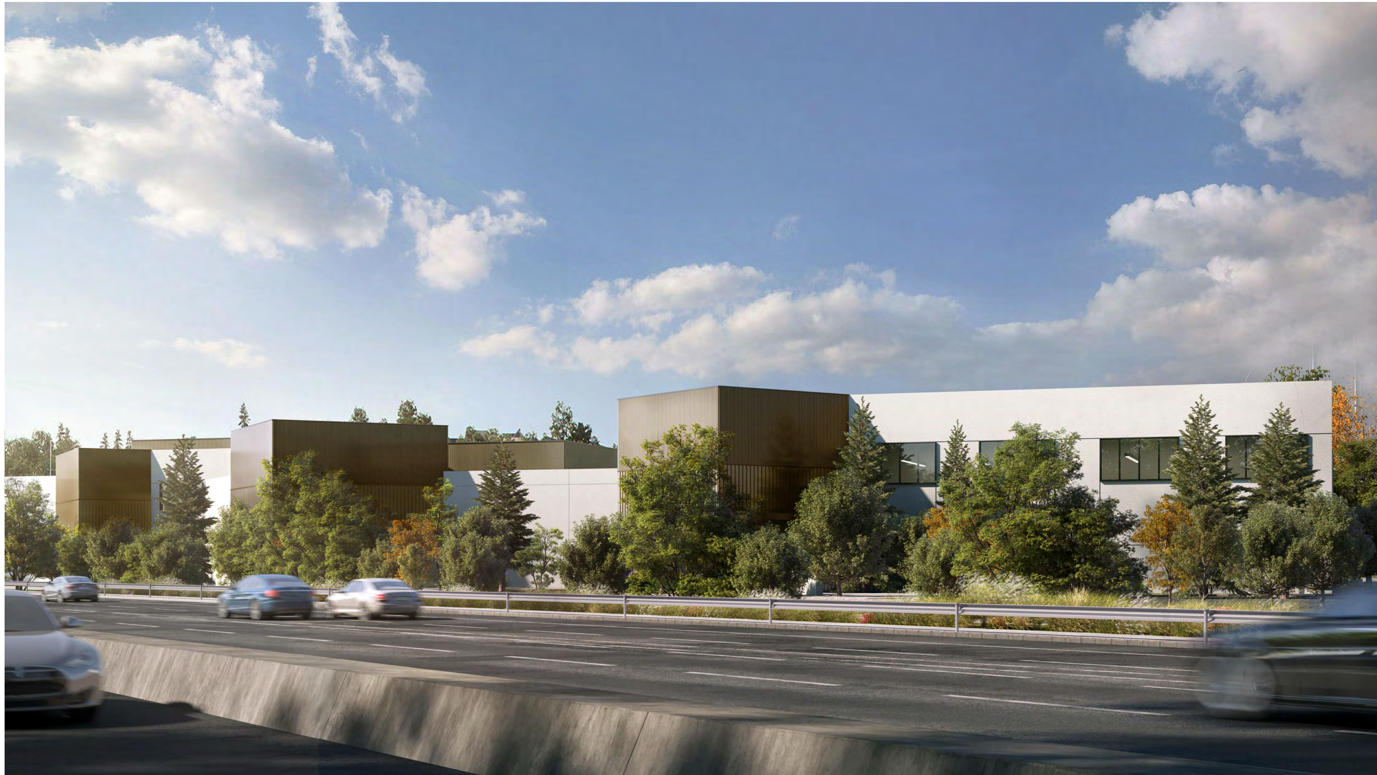
1 VIEW LOOKING SOUTHEAST FROM THE 101 AT THE REAR OF THE PROJECT
