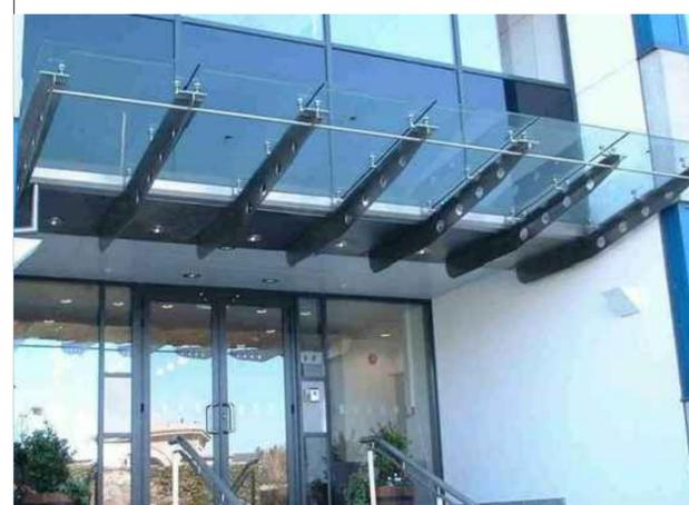
ALUMINUM AND GLASS ENTRY CANOPY - CLEAR LAMINATED TEMPERED GLASS WITH BRACKET SUPPORTS BY CRL, #GAB48. NTS 7
