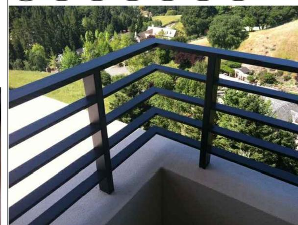
FLAT BAR RAILING SYSTEM BY DECK-RAIL, OR APPROVED EQUAL. NTS 6
