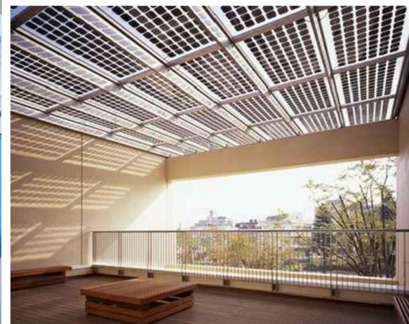
SEMI-TRANSPARENT PV PANELS BY SUN POWER, LG ENERGY, OR APPROVED EQUAL. NTS 7
