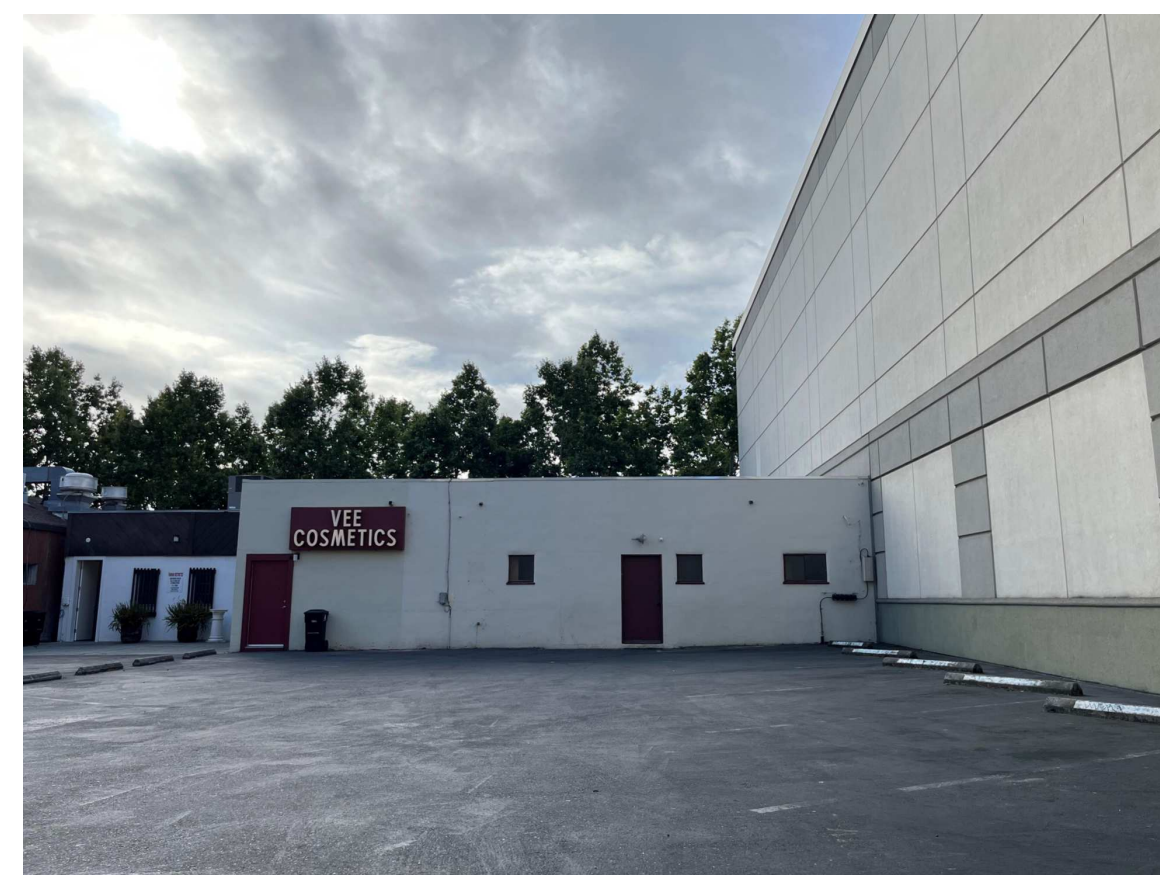
(E) REAR BUILDING VIEW SHOWING ADJACENT BUILDINGS
