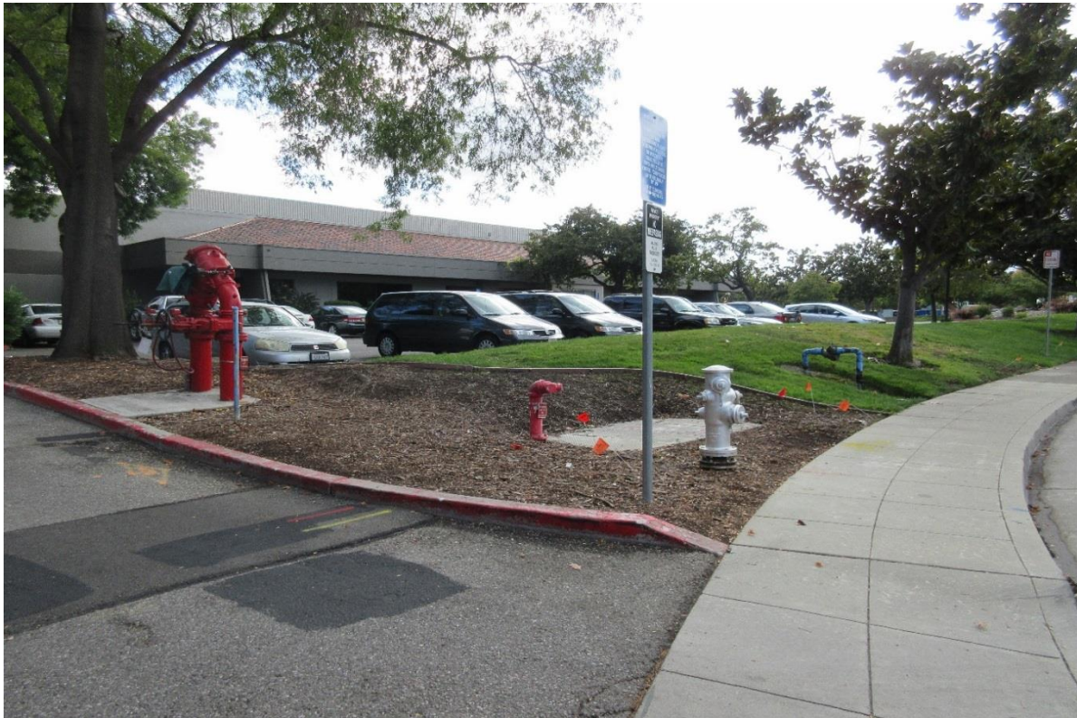
Photo 2: View of the one-story building at 800 East Middlefield Road building, looking southeast.
