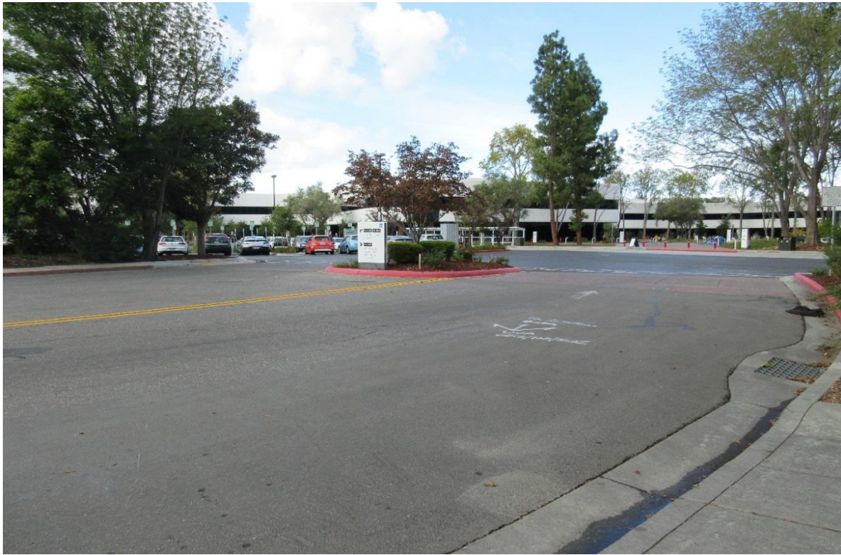
Photo 1: View to the north of the three two-story 700 East Middlefield buildings at the main entrance of the site through the driveway located on East Middlefield Road and North Bernardo Avenue.
