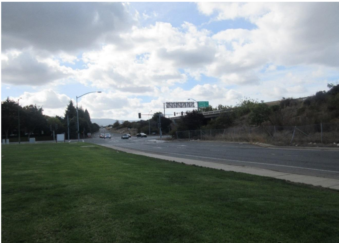
Photo 8: Landscaping in Caltrans easement on project site, view of the SR 237 frontage road and SR 237 to the west of the project site.
