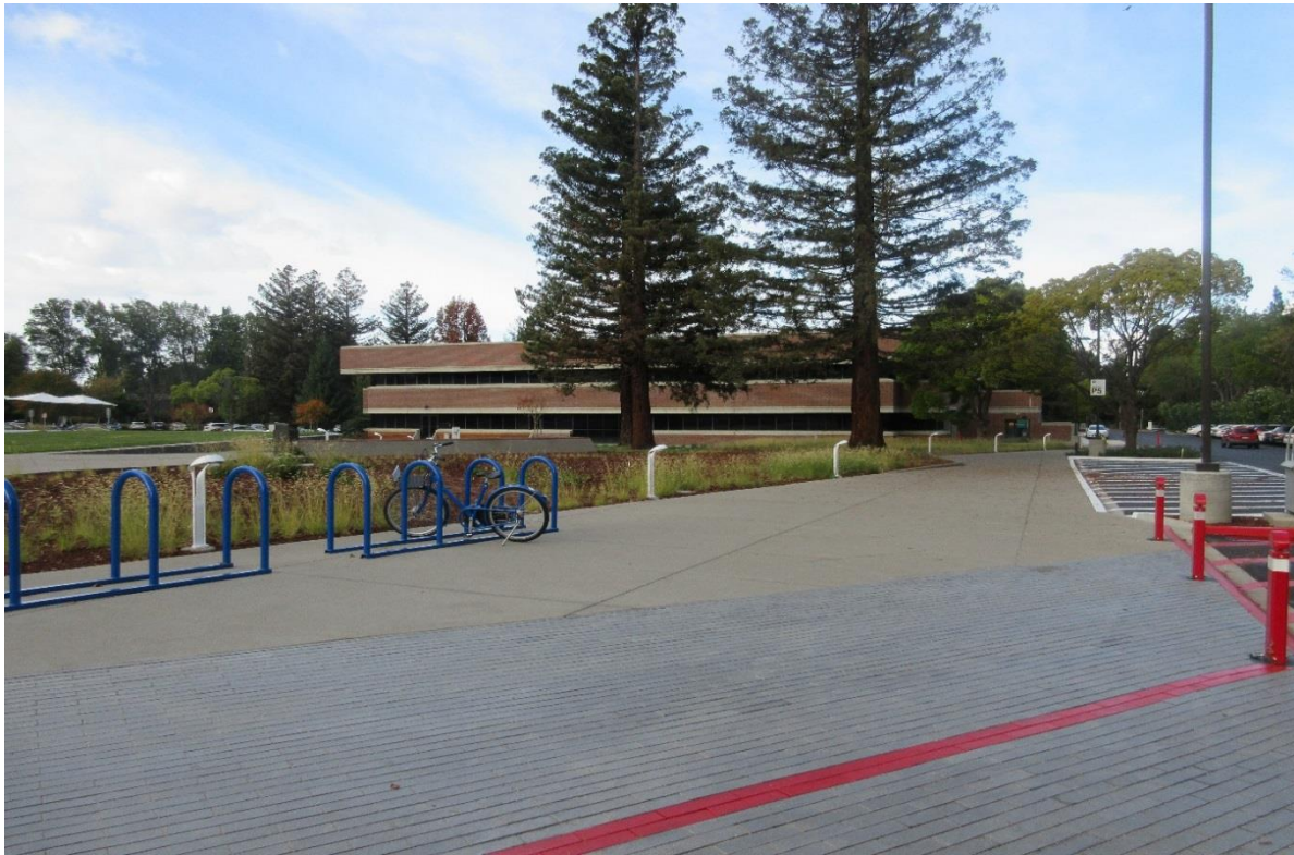
Photo 6: View of the 1101 West Maude Avenue building, looking north
