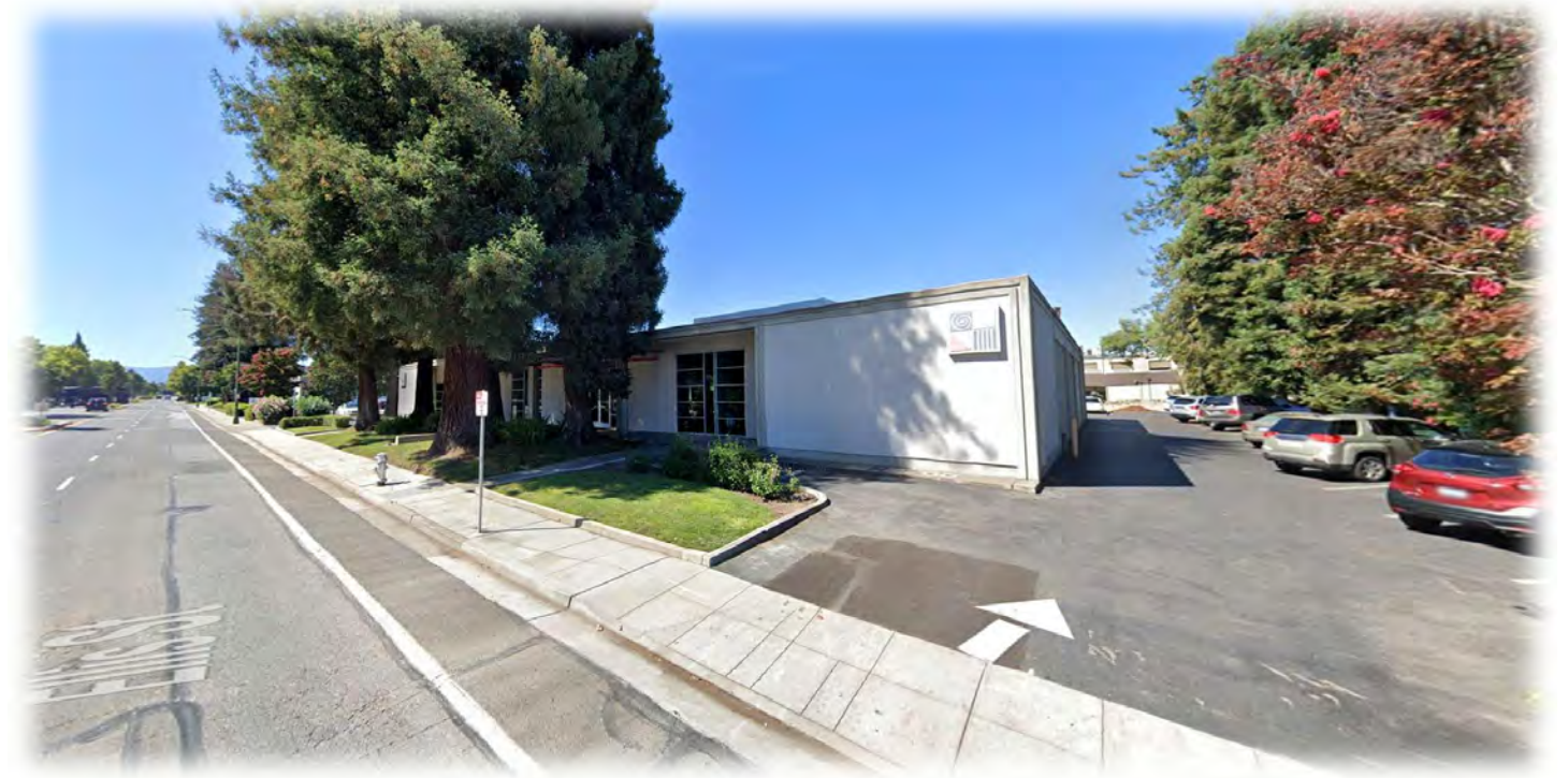
(B) VIEW FROM CORNER OF ELLIS ST. (LOOKING SOUTHWEST)
