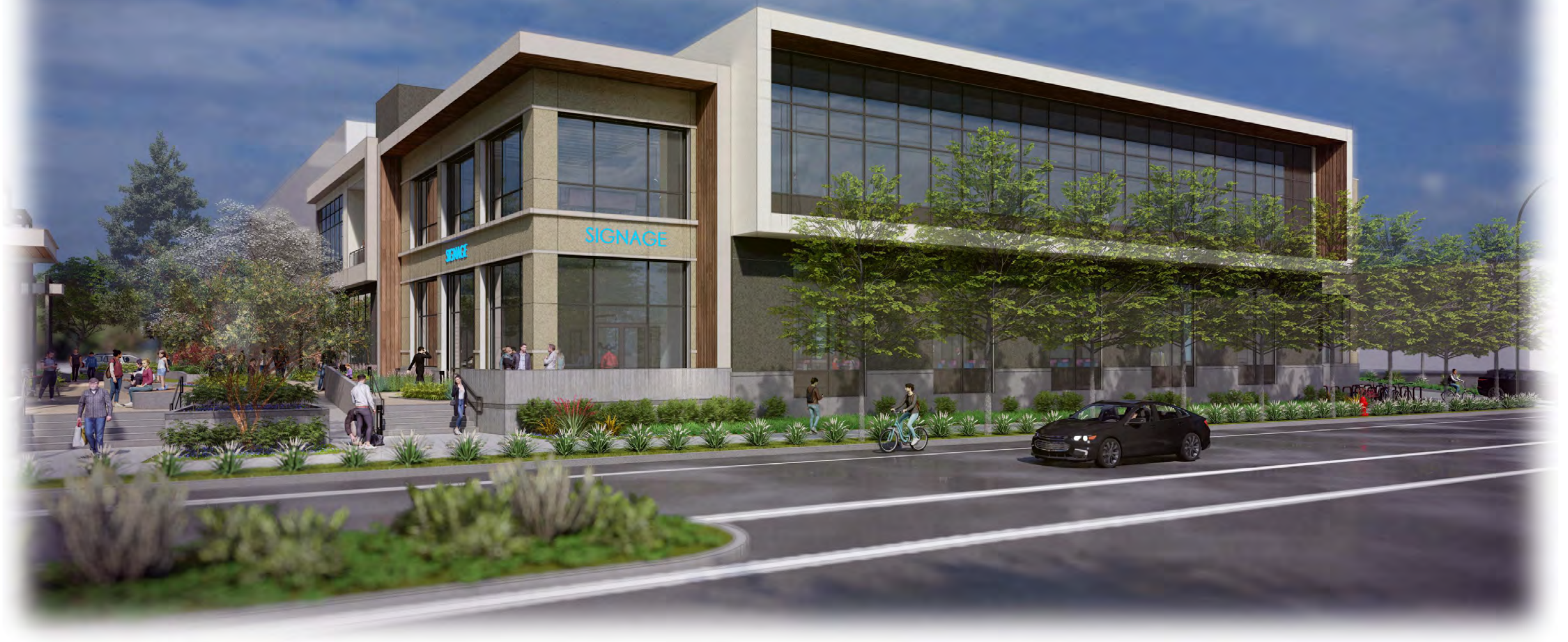
VIEW OF OFFICE FROM ELLIS STREET (NORTHEAST)
