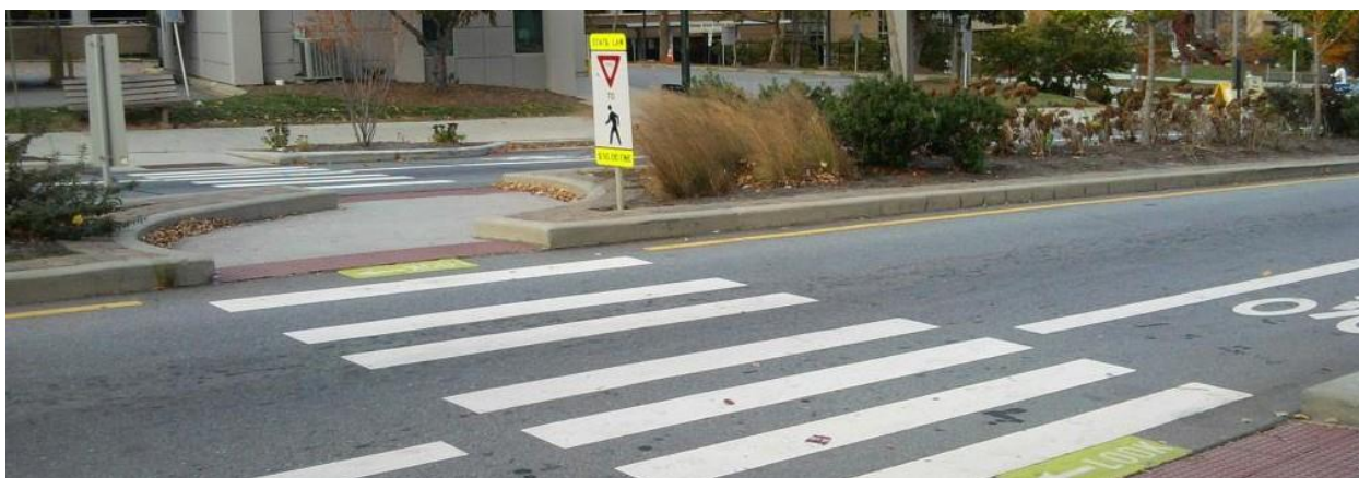
Example of mid-block crosswalk
