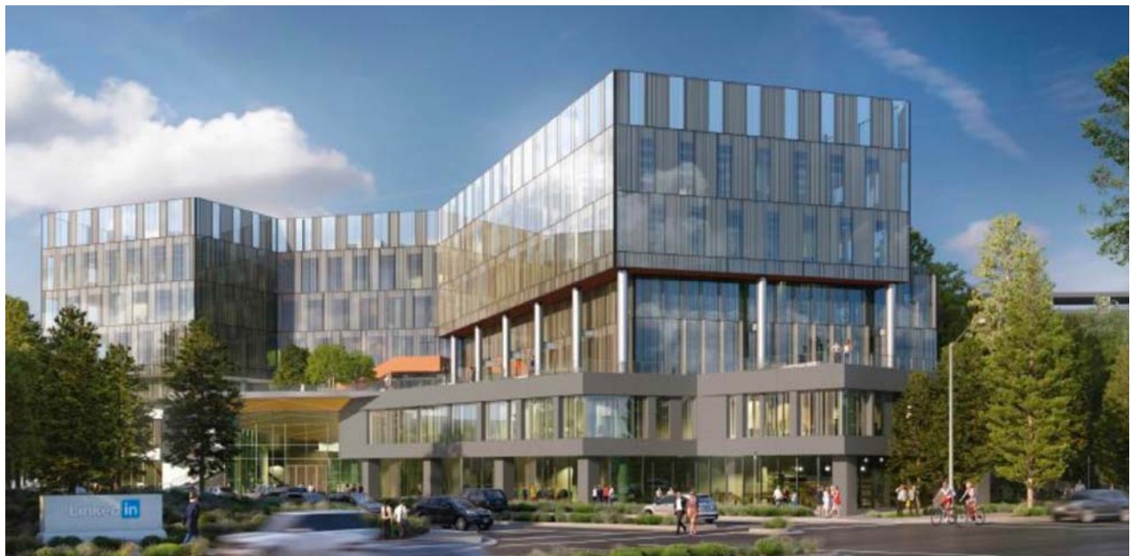
Glass curtain wall with visual interest
