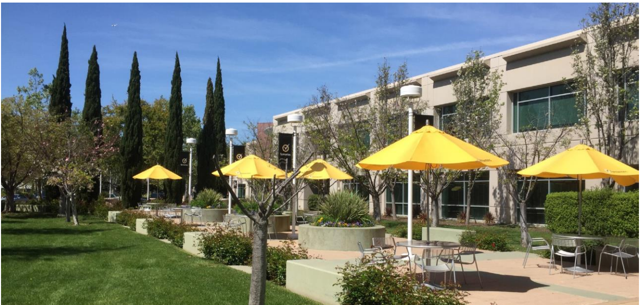
Office campus in East Whisman
