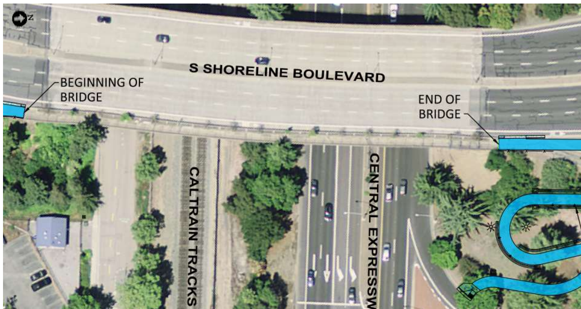
Figure 5: Shoreline Boulevard Overpass Structure
