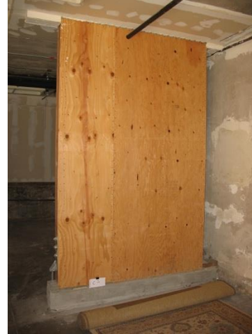
New stand-alone wood shear wall with new concrete footing
