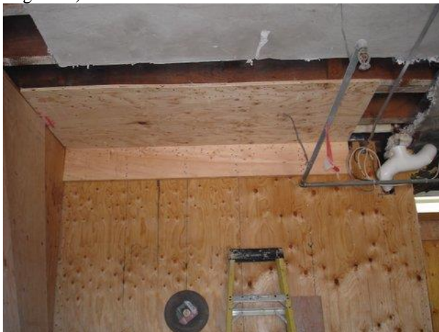
Local strengthening of the second floor diaphragm (Credit: Anthony DeMascole)
