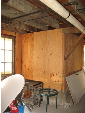
Wood sheathing applied over existing studs, using the existing concrete foundation
