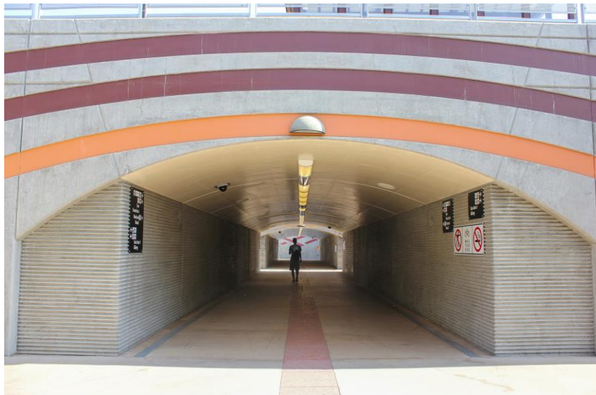
Figure 7: Santa Clara Caltrain Station Undercrossing
