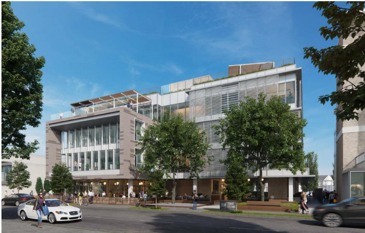
View of Proposed Project from Villa Street
