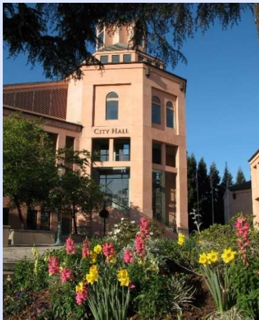
Electrification During Renovations (B4.1)
