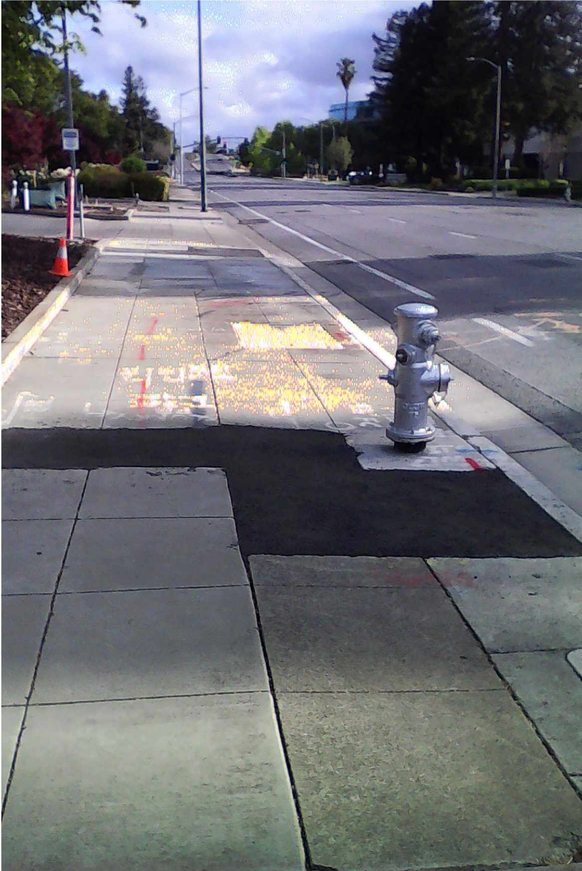
Outside Chevron station -- Sidewalk 4 slabs wide so hydrant doesn't get in pedestrians' way. No setback from street.
