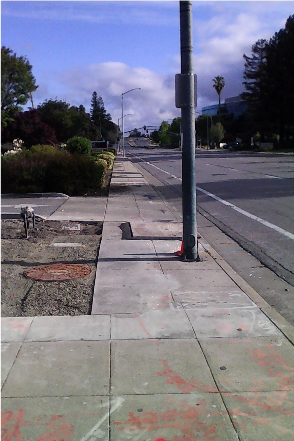
850 Shoreline -- Sidewalk narrows to 6', including curb; no setback. Pole obstructs pedestrians. Shrubbery obstructs view of drivers exiting property. Covering of recent excavation creates tripping hazard.
