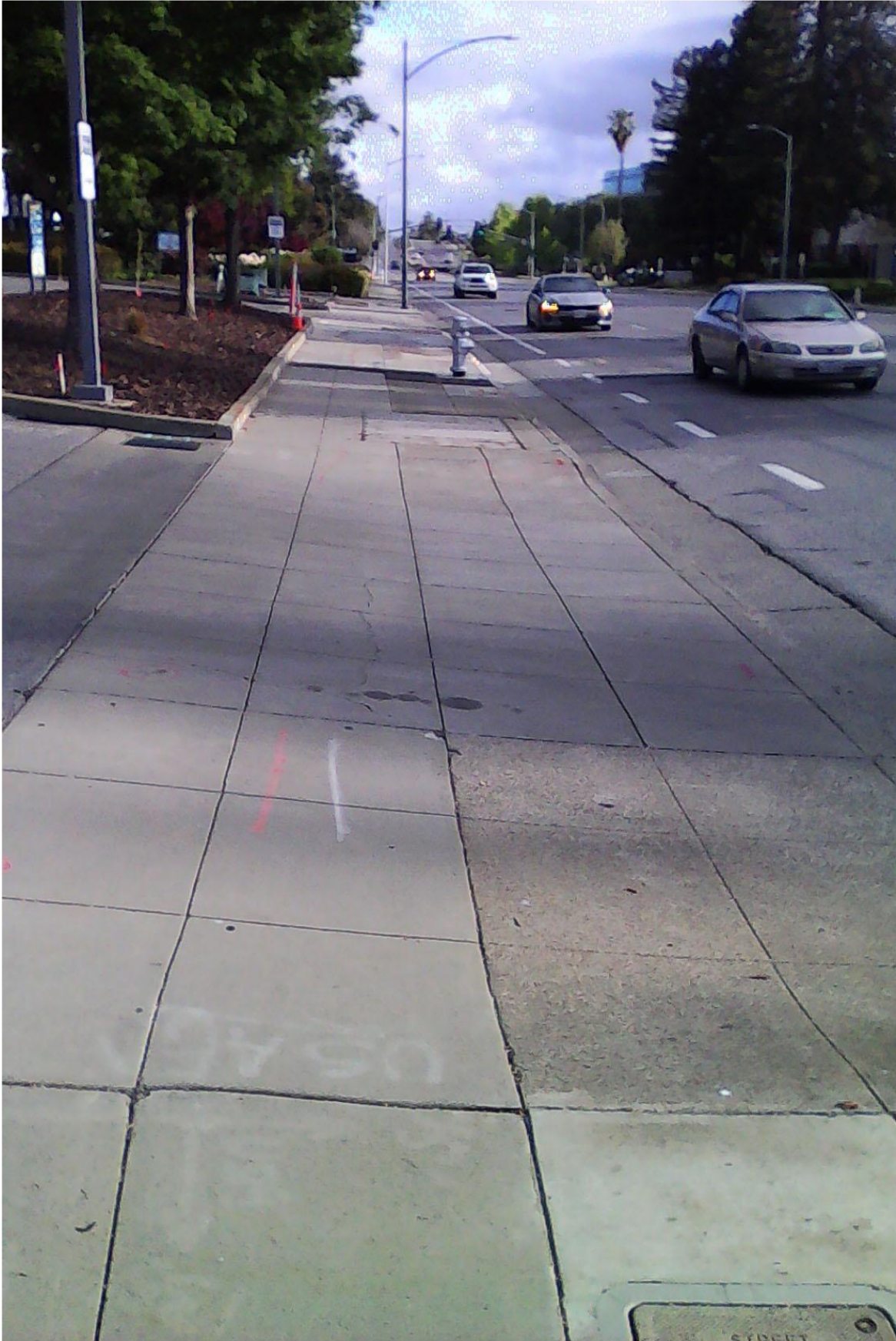
Chevron station south driveway Good place to get run over by driver anxious to exit station
