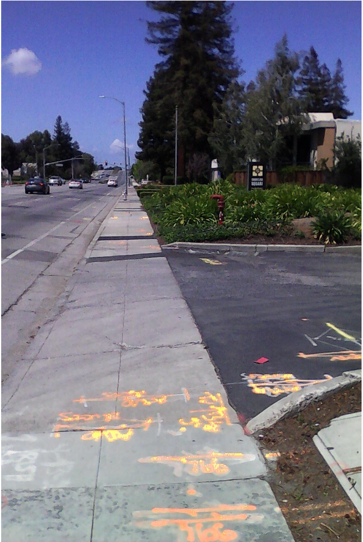
Shoreline Square driveway. One more good place to get run over. Sidewalk ~6', not level, no setback.
