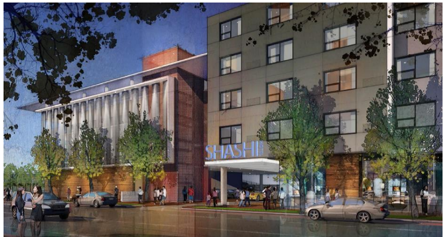
Hotel and Parking Garage Entries Viewed from Space Park Way
