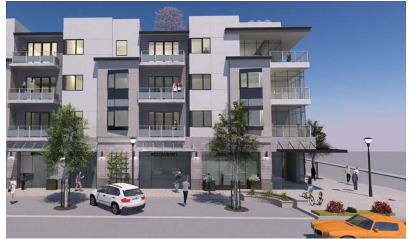
CASTRO AVE - AT CASTRO & FAIRMONT
