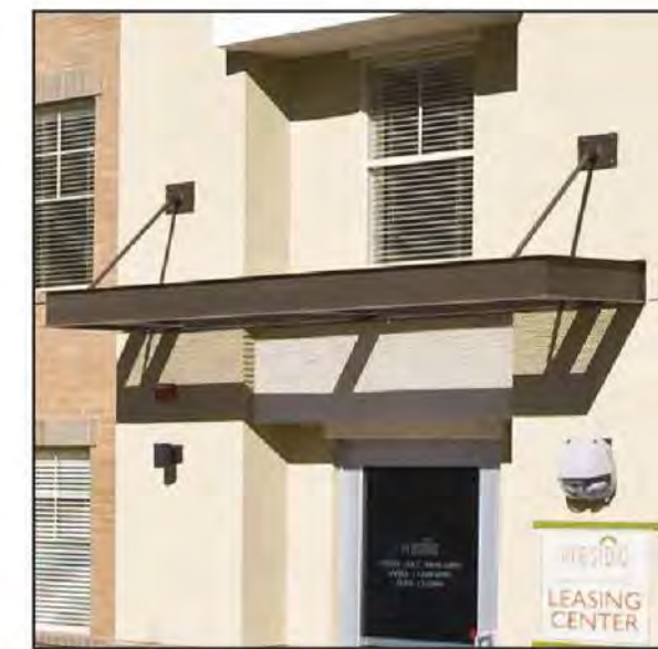
6 PAINTED METAL AWNING W/ TIEBACKS PAINT GRADE
