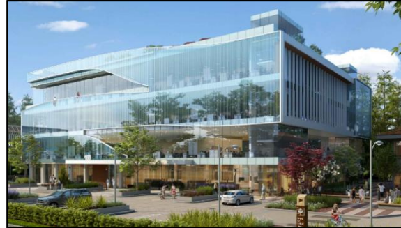
Figure 6: View from North
