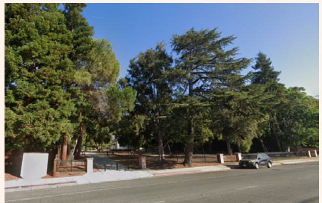
A historical building divides the front of the site from the back, impeding “line of sight” and a sense of safety.
