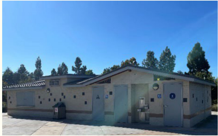
A centrally located and permanent bathroom at Shoreline Athletic Fields.
