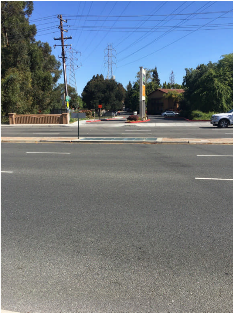
Figure 3-2: Skylight visible at surface of road way median, Stevens Creek Trail tunnel at El Camino Real, Mountain View
