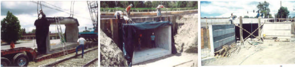
Figure 4-4: Construction Stages of the San Antonio Caltrain Pedestrian and Bicycle Underpass
