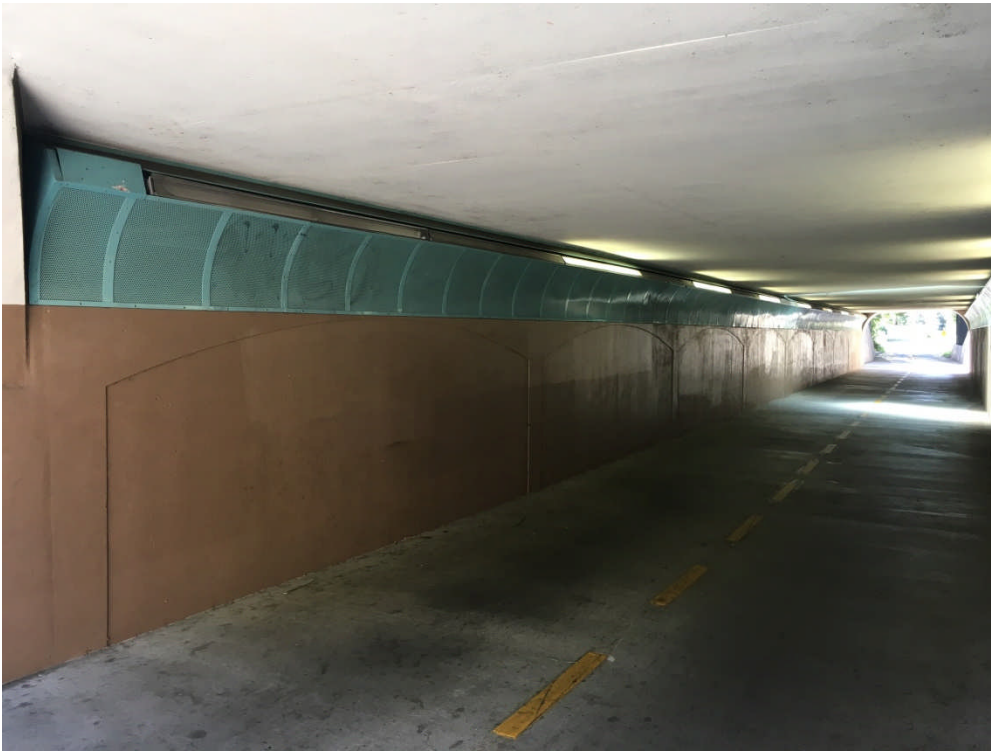
Figure 3-3: Lighting and wall and ceiling colors, Stevens Creek Trail tunnel under El Camino Real, Mountain View
