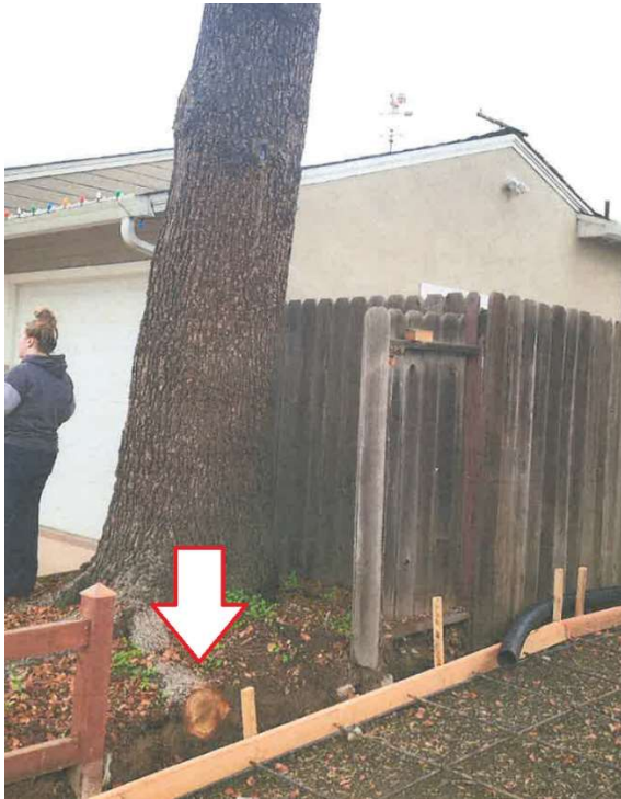
Figure 7: Photo of 7"-8" root cut to repair/replace residence driveway.
