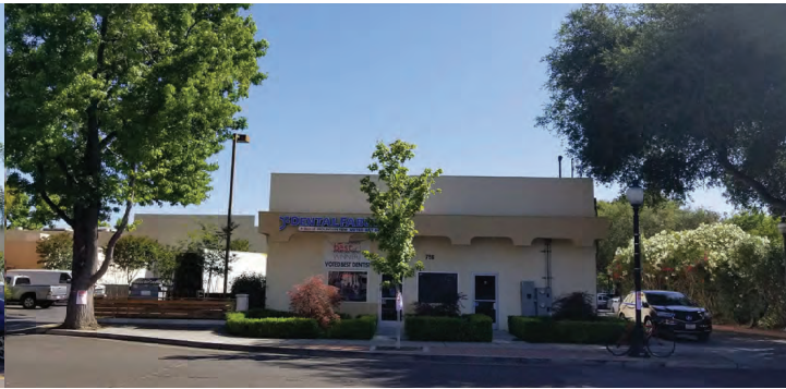
EXISTING PHOTOS AT 756 CALIFORNIA STREET
