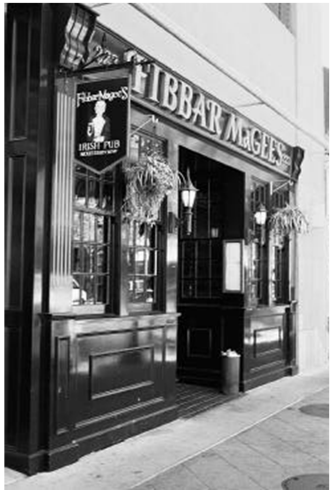
Fig. H.24: New storefront renovation on Castro Street. Entrances should be recessed from the facade, creating a small alcove.
