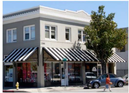
Fig. H.7: Canopies help provide a pedestrian scale to the building.
