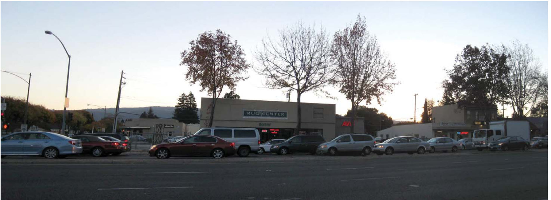
1. View looking south of existing El Camino Real site frontage.
