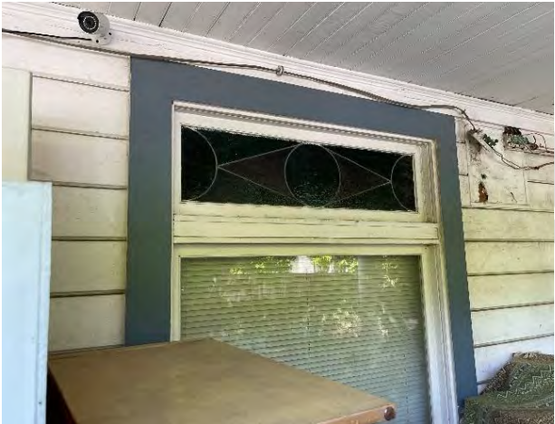
Figure 3. Porch window with leaded glass transom, view southeast.
