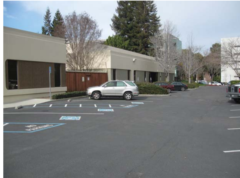
2. View showing the two single-story buildings located at 580 and 620 Clyde Avenue.
