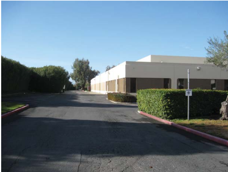
1. Looking west along southern boundary of the project site, showing the single story building located at 580 Clyde Avenue.
