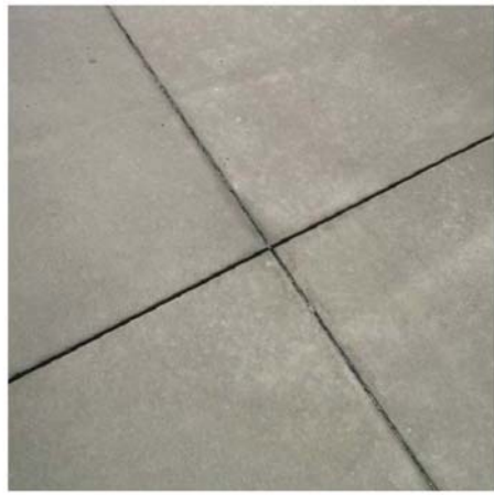
Scored Concrete Paving
