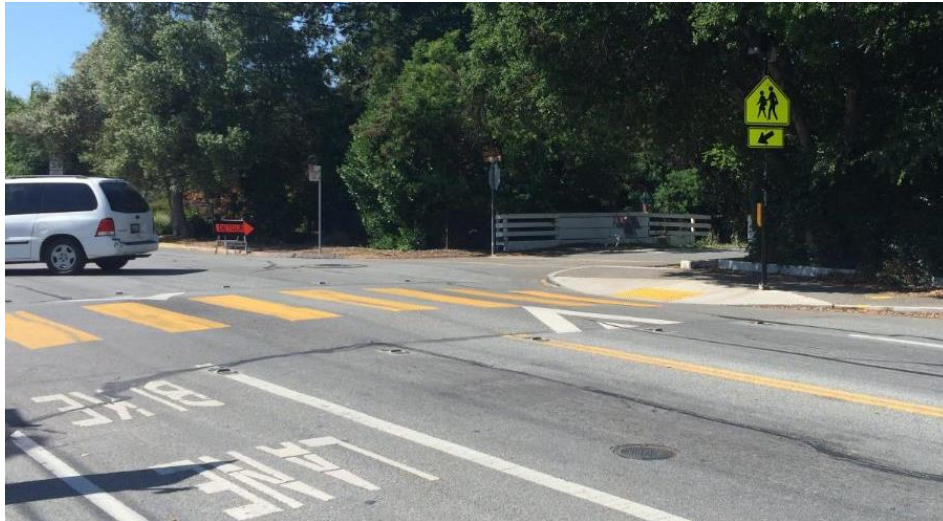
Figure 4 – Example of a Raised Crosswalk
