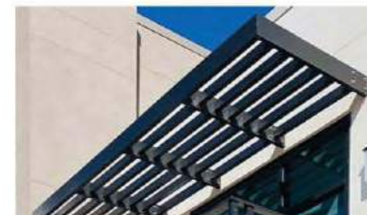
M1 METAL SOLAR SHADE - AVAEK ANODIZED ALUMINUM - DARK BRONZE
