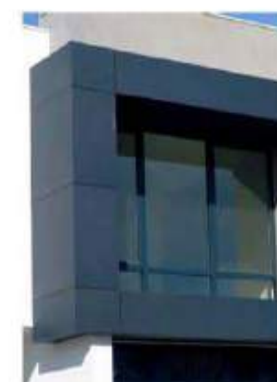
A1 ALUMINUM CLADDING AT CANOPY - ALUCOBOND - BONE WHITE
