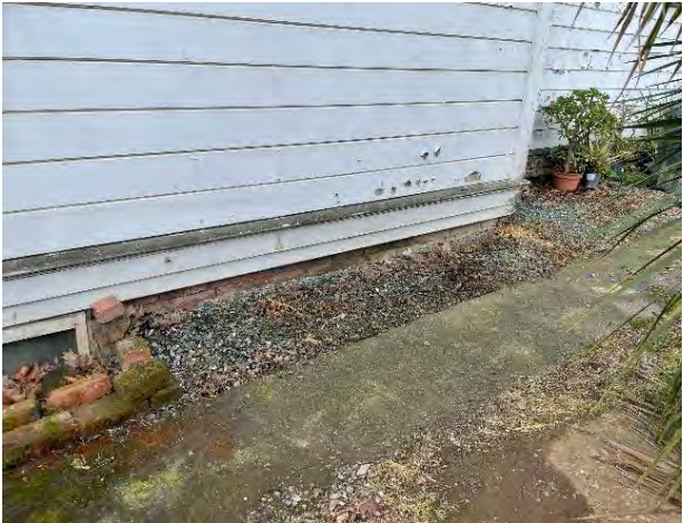
Figure 5. Brick visible at foundation of north facade, below cross-gabled portion, view southwest.
