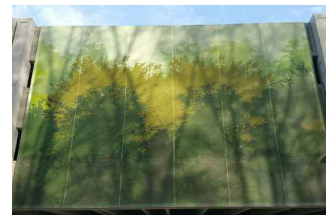
(PS) TENSILE MESH FAÇADE SCREEN, STRUCTURFLEX FABRIC : COATED PES MESH - SERGE FERRARI SOLTIS FT 381 FRAME : FACID 65 ALUMINUM FRAME
