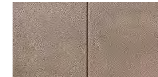
On Structure Paving
