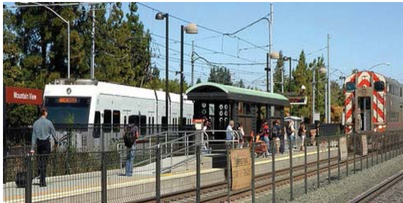
Caltrain and VTA Light Rail.
