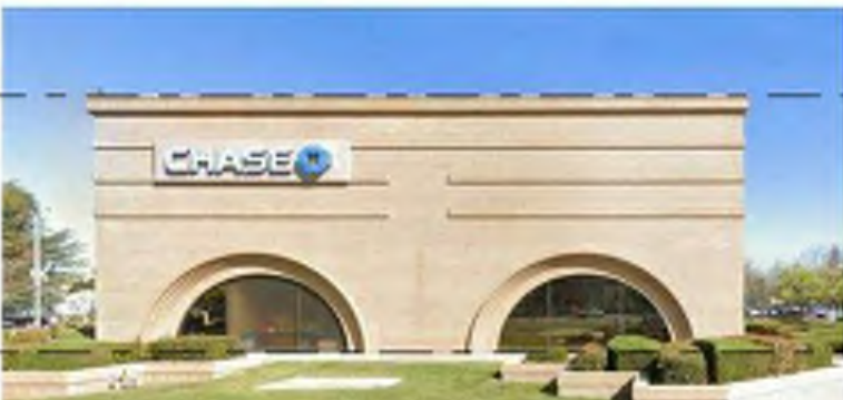
EXISTING CHASE BANK (REMOVED) - SIDE
