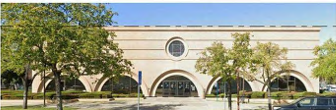
EXISTING CHASE BANK (REMOVED) - BACK
