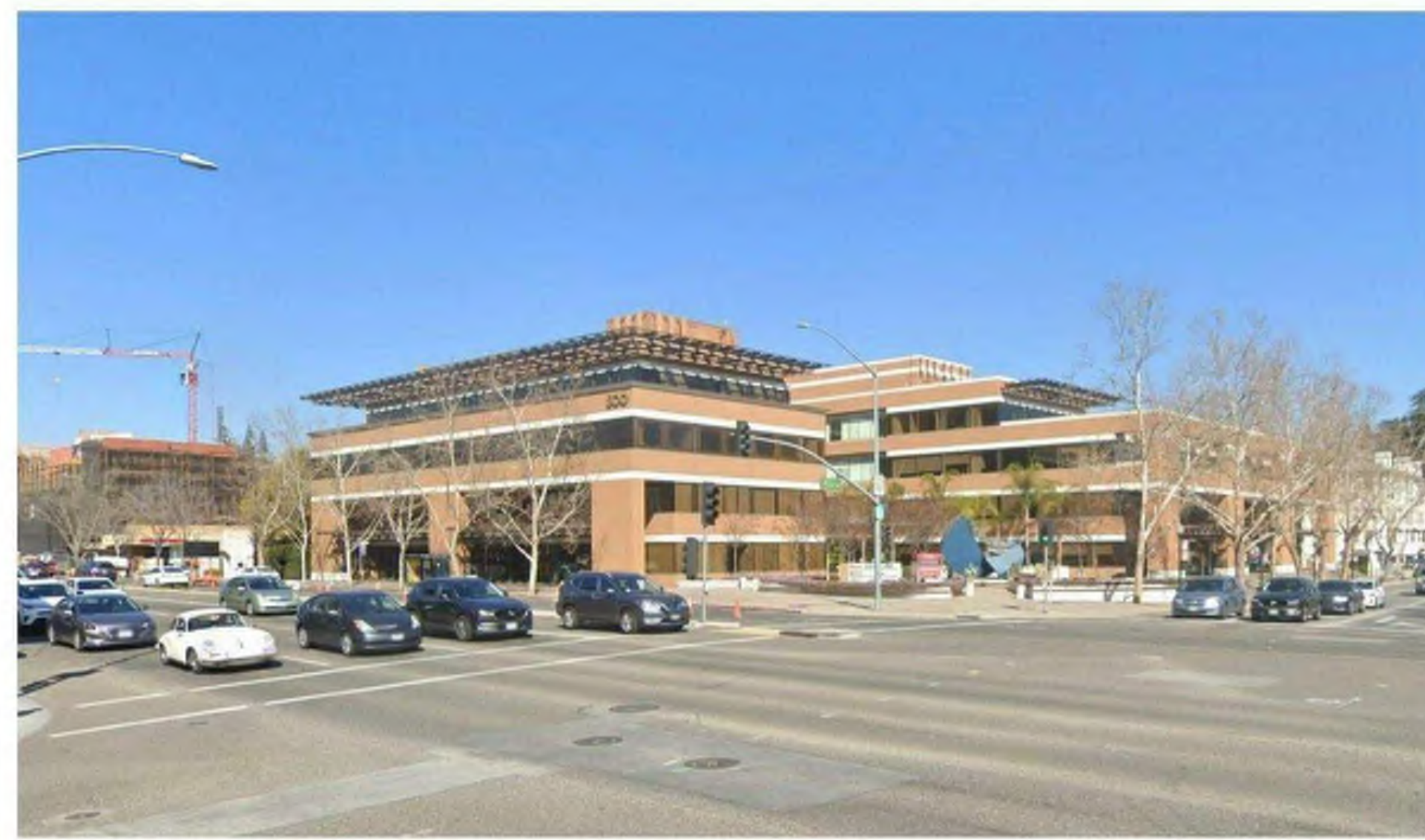
2. OFFICE ACROSS ECR & CASTRO ST INTERSECTION
