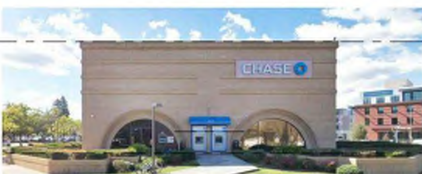
EXISTING CHASE BANK (REMOVED) - ATM SIDE
