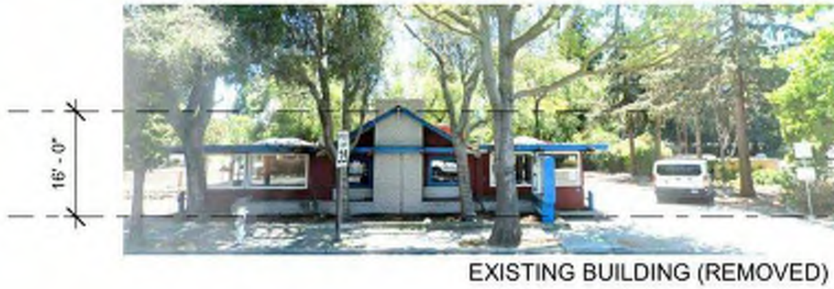
EXISTING BUILDING (REMOVED)
