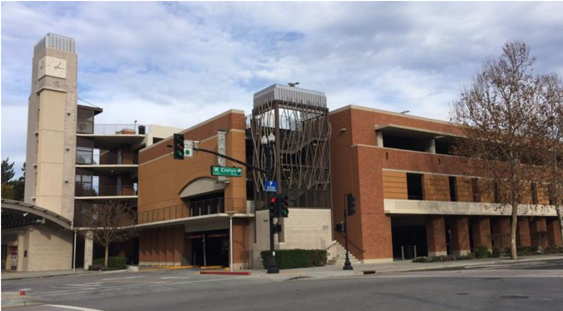
Figure 11 – Sunnyvale Caltrain Station Parking Structure
