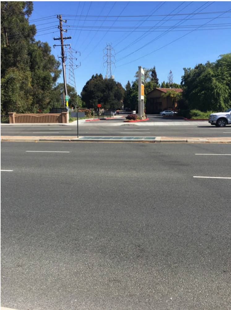
Figure 3-2: Skylight visible at surface of road way median, Stevens Creek Trail tunnel at El Camino Real, Mountain View
