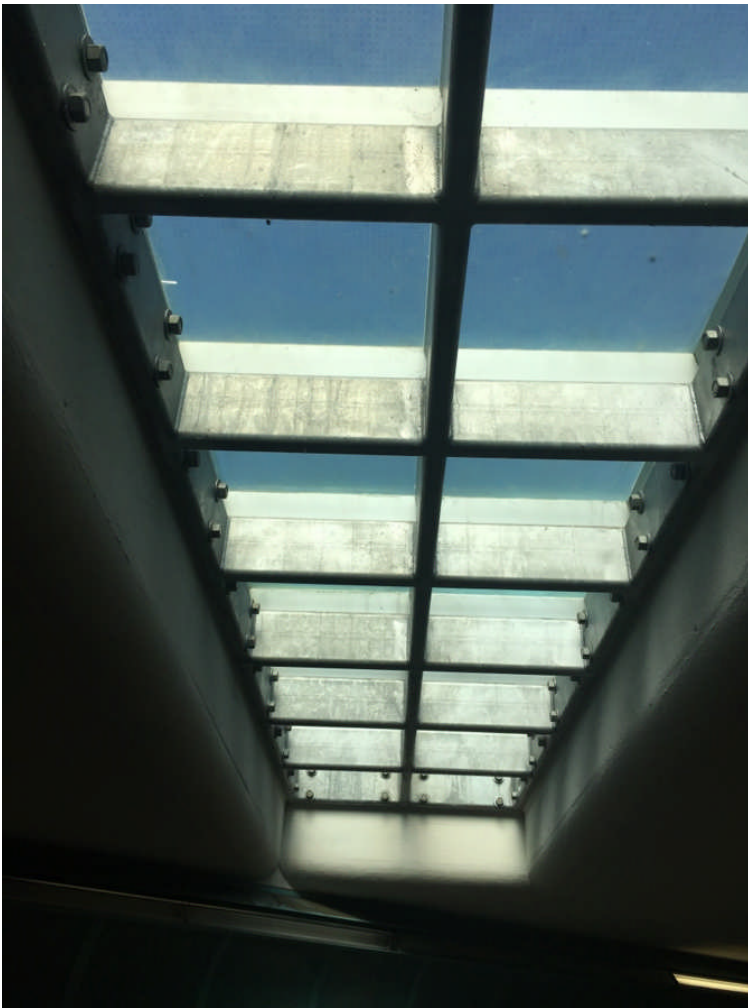
Figure 3-1: Skylight, Stevens Creek Trail tunnel under El Camino Real, Mountain View
