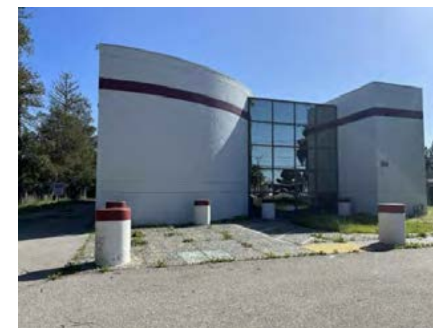
10 - EXISTING STRUCTURE - LOOKING SOUTH AT CENTER OF SITE
