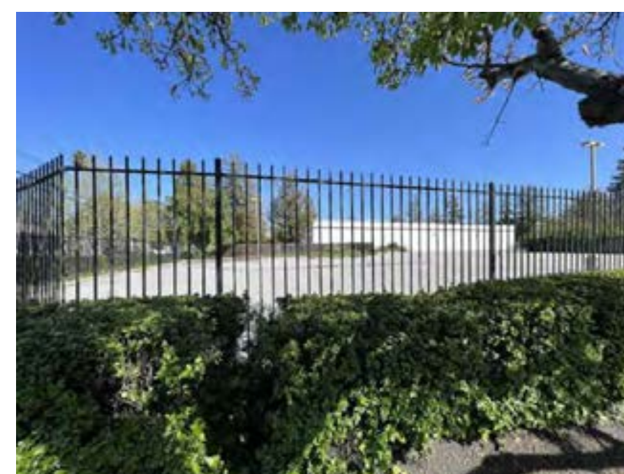
13 - STREET VIEW - INDEPENDENCE AVE - EXISTING FENCE + LANDSCAPING ON SITE - LOOKING EAST
