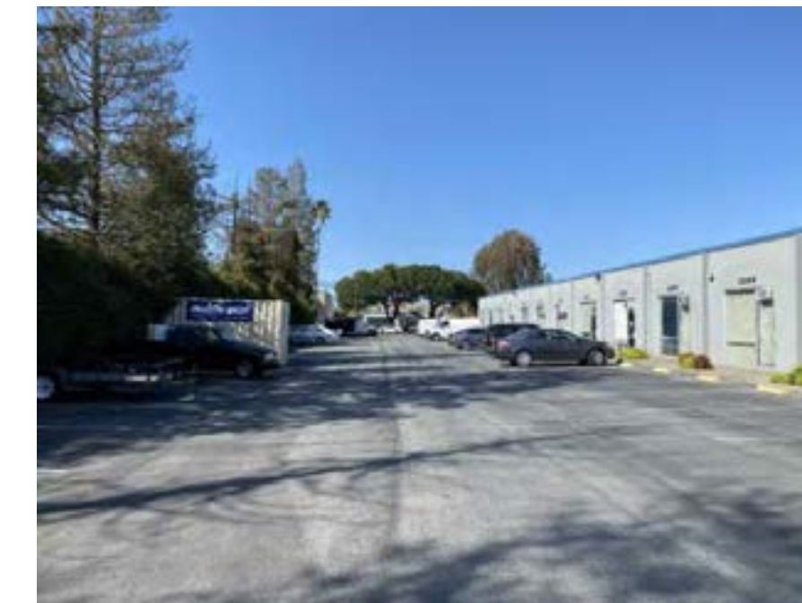
6 - EXISTING STRUCTURES - LOOKING NORTH FROM CENTER OF SITE
