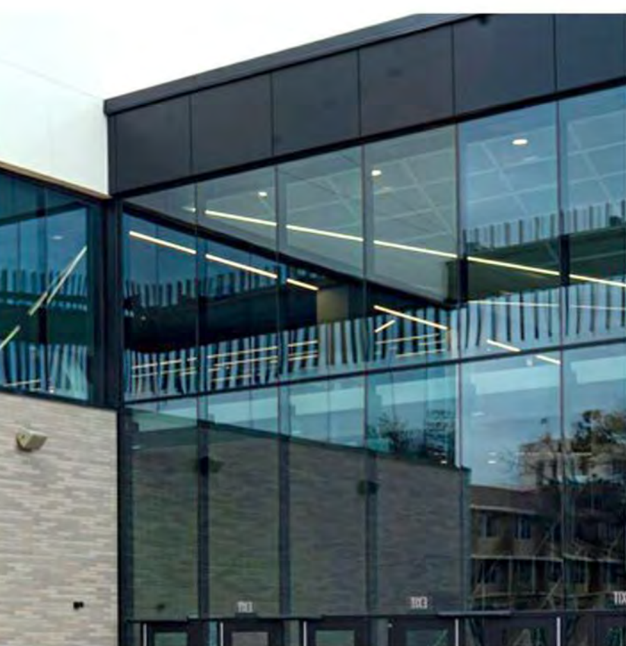
C1-2 BUTT JOINT GLASS SYSTEM MULLIONS SIT BEHIND GLAZING WITH TINE, WALTERS & WOLF OR EQ., PAINTED DARK GREY
