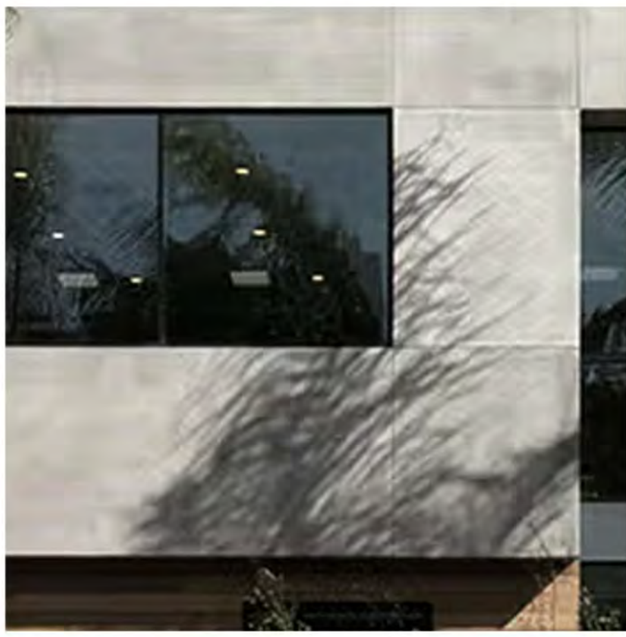
A1-2 STUCCO GREY, APPLIED OVER EXISTING CMU WALLS
