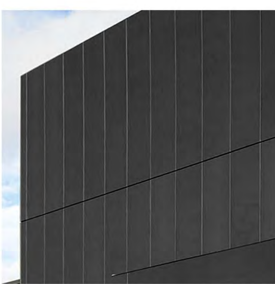
B1-4 ALUMINUM PANEL RAINSCREEN NORTHCLAD OR EQ.ACM RAINSCREEN PANEL , CONCEALED FASTENERS, LEXUS BRONZE
