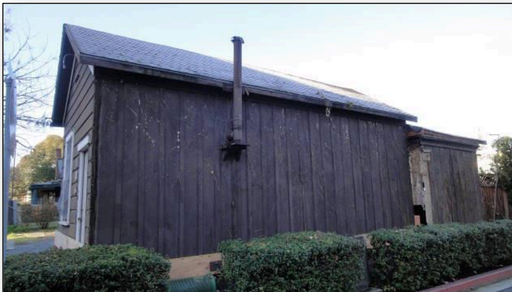
Figure 2 – Immigrant House in its original location at 166 Bryant Street. Looking south at the side of the building.
