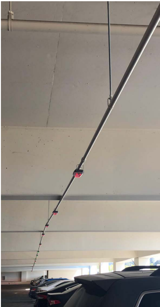
Image 258. Parking Sense Overhead Sensors
