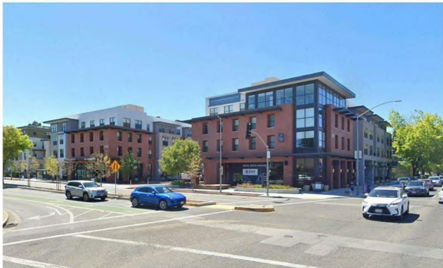
1. APARTMENT @ CASTRO ST & ECR INTERSECTION
