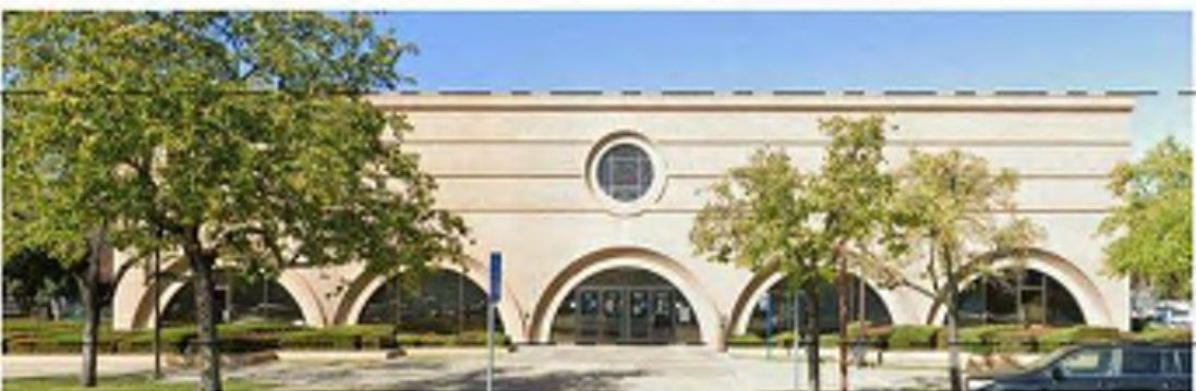
EXISTING CHASE BANK (REMOVED) - BACK
